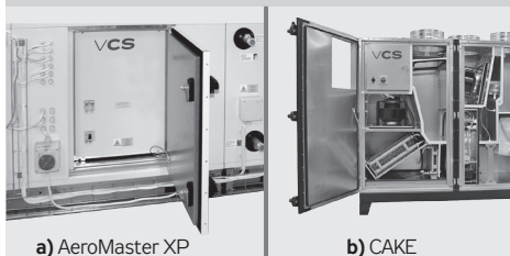
Figure 2 – installation inside air handling unit
